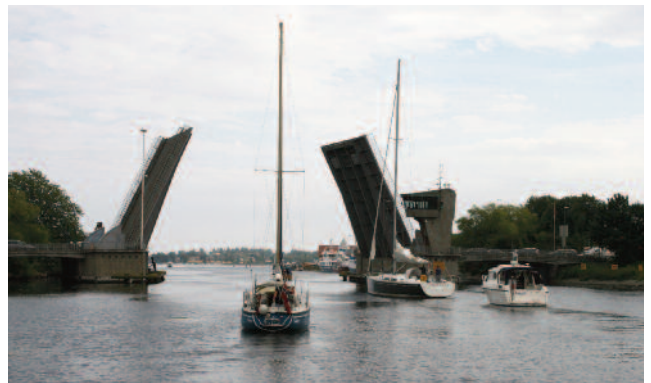
Tønsberg bridge opening
